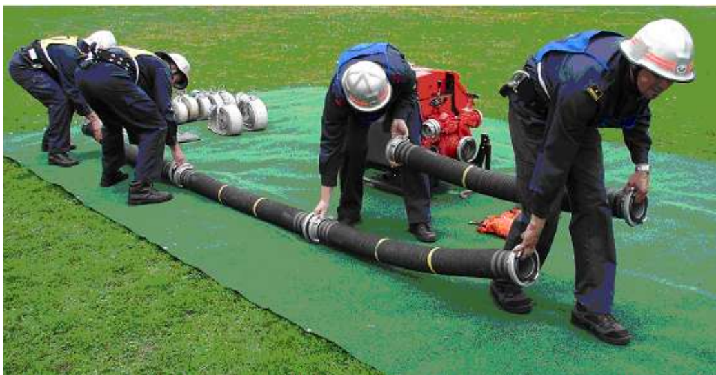
Fig. 4b: Laying-out the suction hose by the HTR
